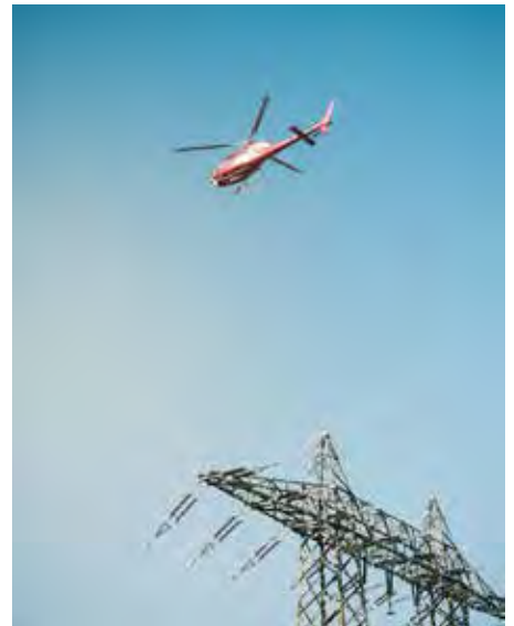
Helicopter testing of electricity lines.
